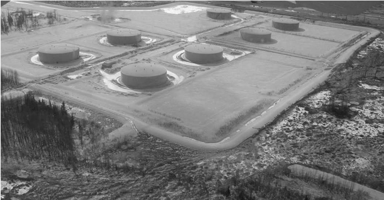
March 28, 2009 - Mud torrents triggered by Mt. Redoubt's eruptions reach the top of the protective dike around storage tanks at the Drift River Terminal, and in some places have lapped over the top.
